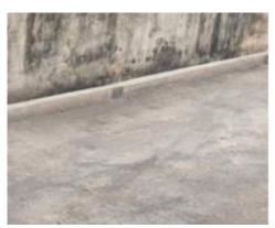
Built brick barricade to avoid resin flow into drain
