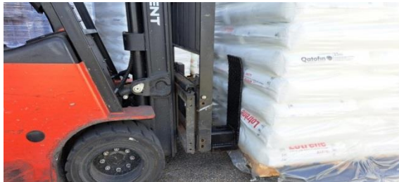
Installation of forklift stopper to avoid stabbing the material bag
