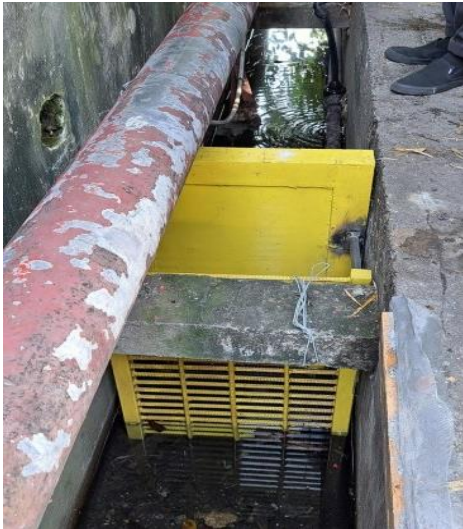
Installation of filters in water drainage
